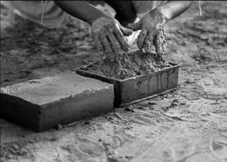
One standard room in the camp is usually 2m x 3m, requiring 1,000 bricks. A woman can make an average of 100 bricks a day. These mud bricks are an environmentally friendly alternative to the more common red bricks, which need to be fired. However they are not as durable.
