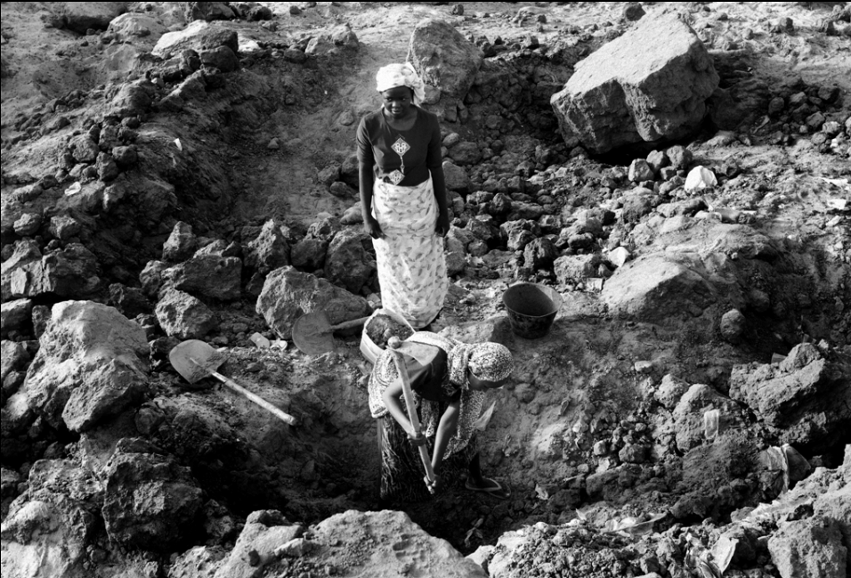
One standard room in the camp is usually 2m x 3m, requiring 1,000 bricks. A woman can make an average of 100 bricks a day. These mud bricks are an environmentally friendly alternative to the more common red bricks, which need to be fired. However they are not as durable.
