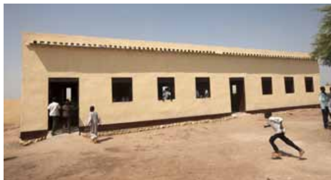
On 3 September 2013 in Shangil Tobaya, North Darfur, students celebrate the opening of the new Secondary School for Girls built in UNAMID's community-based, labour-intensive projects (CLIPs) programme. Photo by Hamid Abdulsalam, UNAMID.
