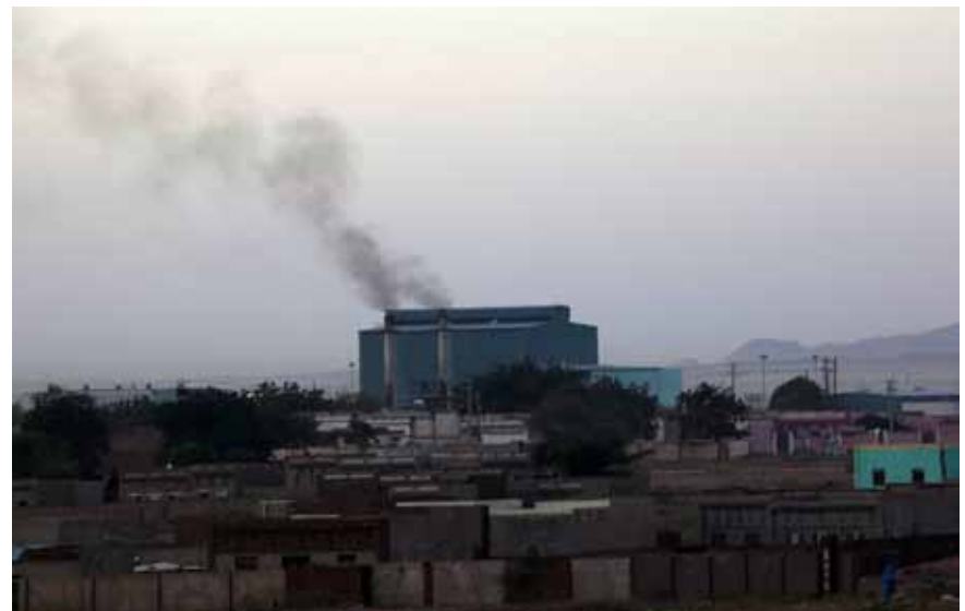
Pictured here is the power plant in El Geneina, West Darfur, which supplies electricity to the entire town. According to the Mr. Haider Gali-Koma, Governor, West Darfur, this plant is likely to be connected to the national electrical line. However, the plant currently uses large electric generators and solar panels to provide electricity. Photo by Hamid Abdulsalam, UNAMID.
