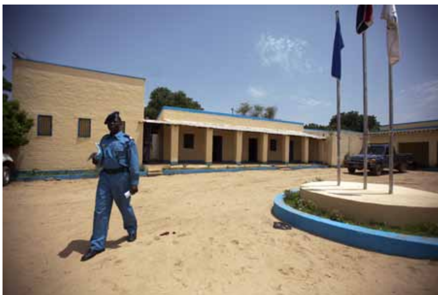
In El Geneina, West Darfur, a Sudanese Police Officer walks outside the courtyard of the new El Geneina detention centre that was recently renovated and expanded through the work of a UNAMID-funded quick-impact project. Photo by Albert González Farran, UNAMID.
